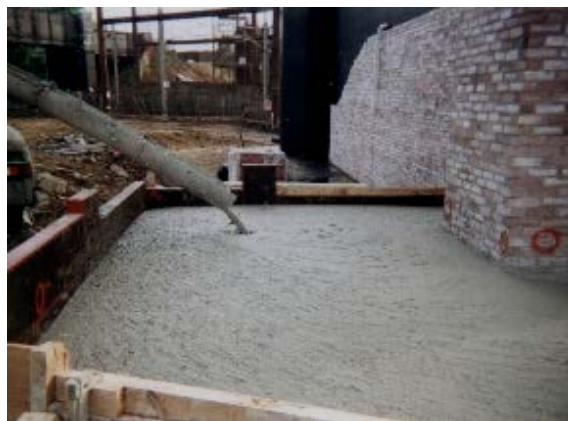
Figure 2: Placement of foamed concrete with the use of removable shuttering
