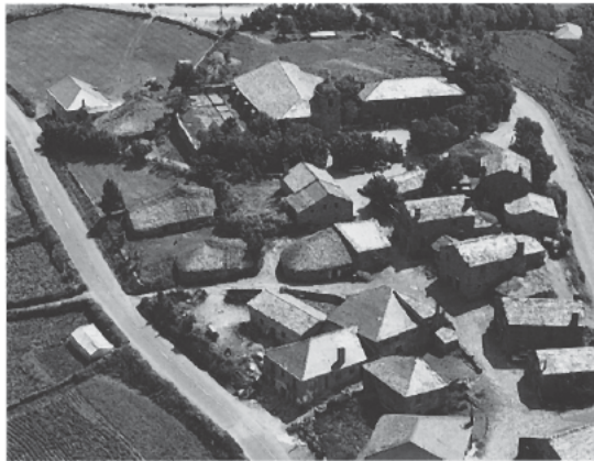
Figure 3. The modern village of O Cebreiro, Galicia. Fotographia de Fama Vigo S.L.
