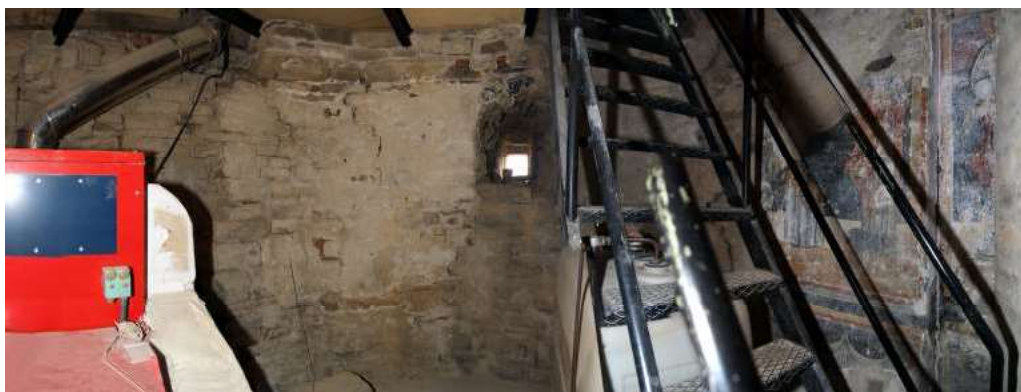
Fig. 4. Vista general interior
