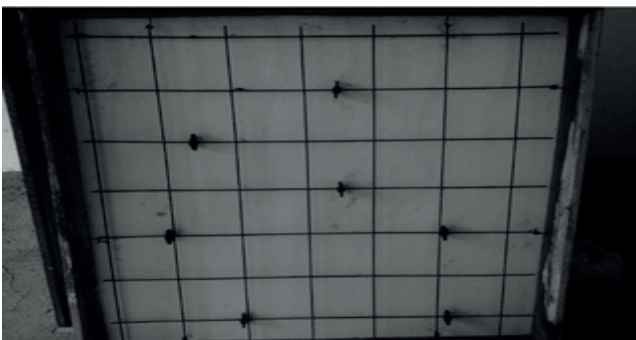
Figure 5. Reinforcement prepared inside the form before casting.
