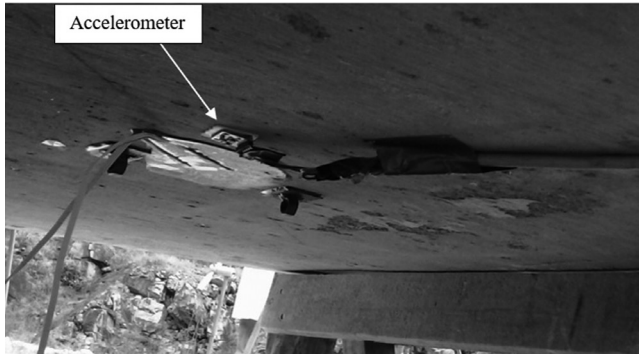
Figure 8. Accelerometer attached to the bottom of the slab before test. Source: Authors
