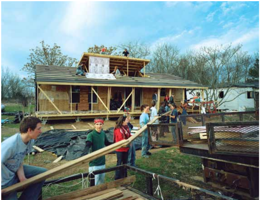
Figure 18. Rose's Courtyard during the building process. Photograph: ©Timothy Hursley.
