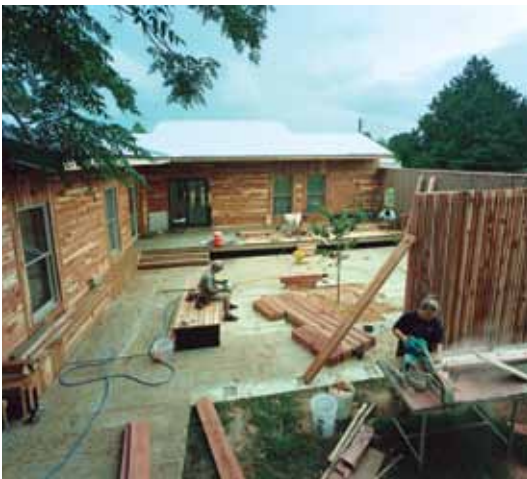
Figure 14. Rose's House during the building process. Photograph: ©Timothy Hursley.
